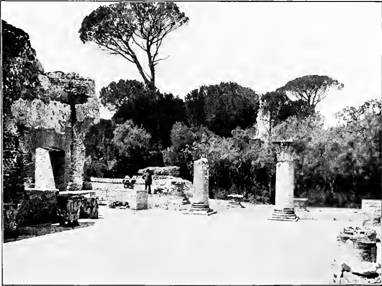
A hall near the Greek and Latin libraries, excavated by the author in 1885
